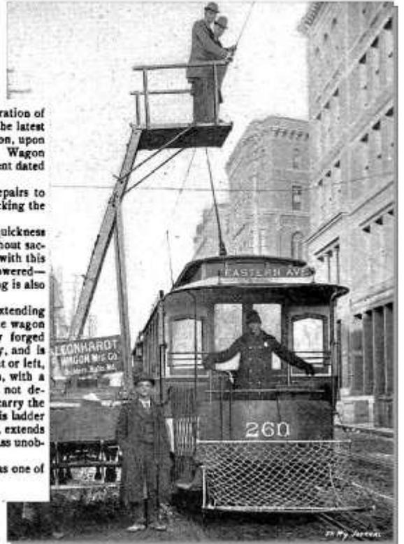
FIG. 3.—TOWER WAGON IN USE WITHOUT INTERFERING WITH CARS.
